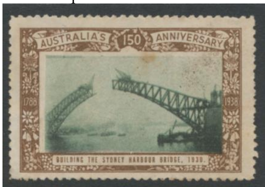
C7/R3 Building the Sydney Harbour Bridge 1930
